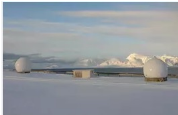
Satellite Receiving Station Ny-Ålesund
